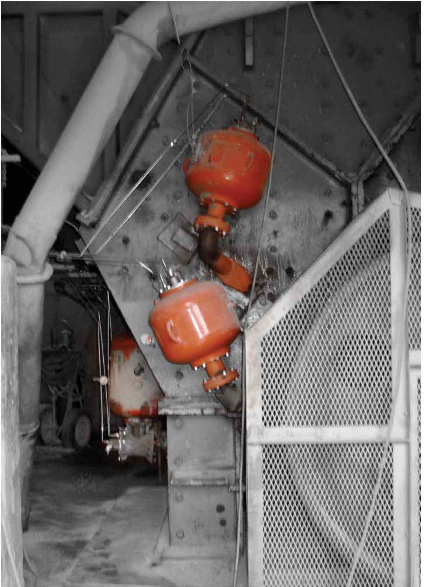
▲ Martin Flow Aids help remove accumulated material and completely empty stacker tubes.
